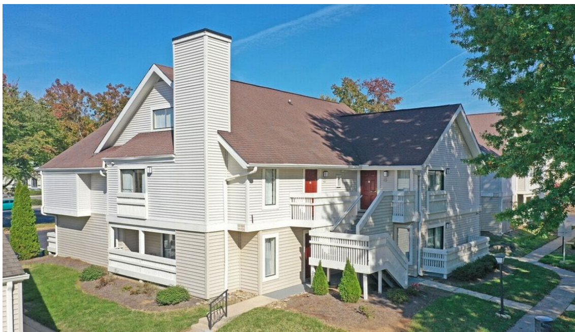
Exterior of Residence Inn building #1 Source: National Association of REALTORS® and Move, Inc
