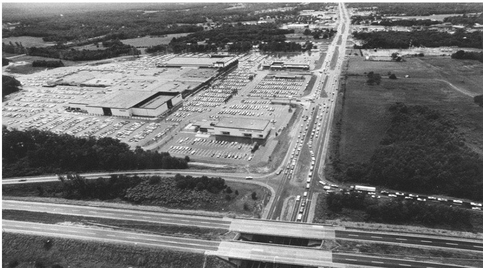
Aerial photograph on the day of the Cloverleaf Mall grand opening in in 1972. Source: Richmond Times-Dispatch
